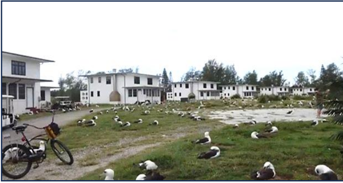
Former WWII bunkhouses
