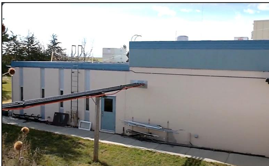
WWV feedlines exiting station
