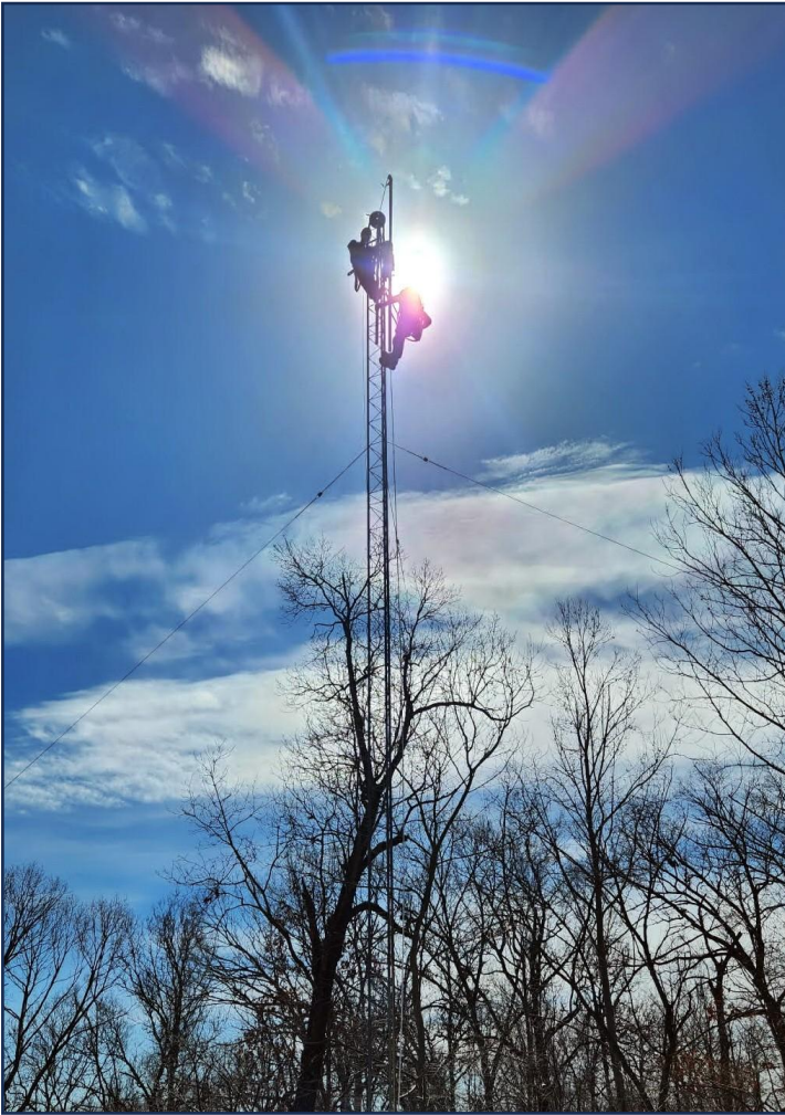
With antennas now removed from the tower, KM5G and N5KWL prepare to lower the first section
