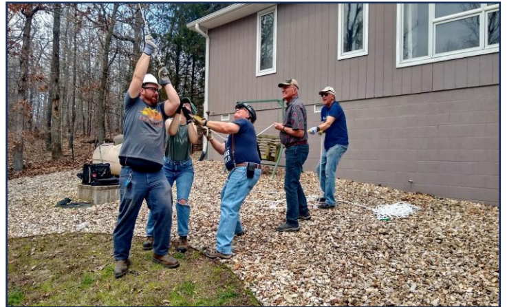
The ground crew lowered each section with a gin pole and pulley
