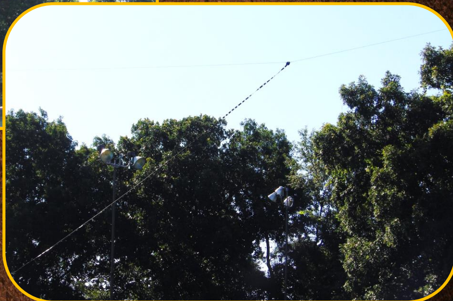
The Digital station's G5RV dipole ▶
