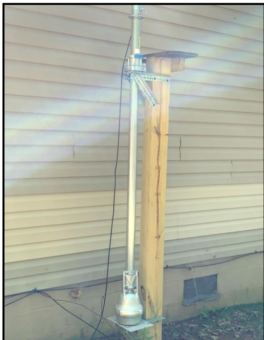
The W5KMK antenna mast in rotator with the thrust bearing above – ground mounted (nifty!)
