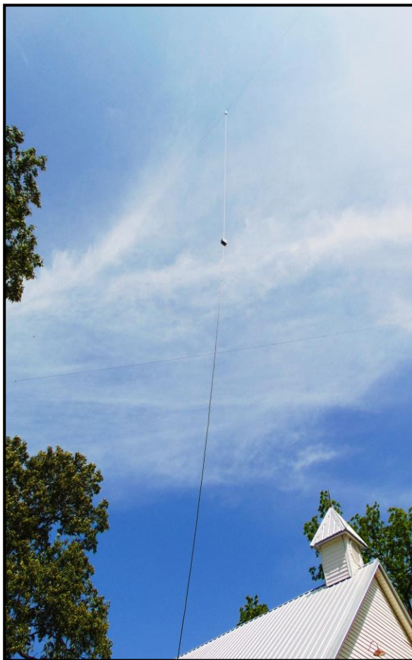
One of two Windom dipoles at 70 feet
