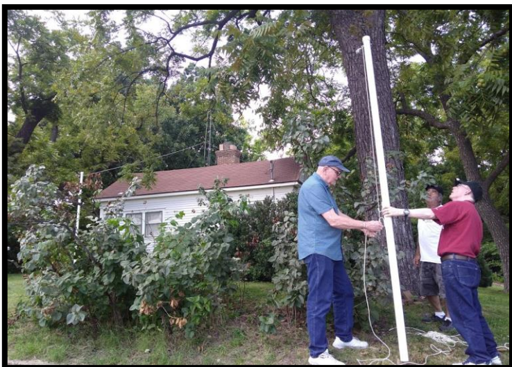
Mark-K5XH, Alan-KEØQFO, and Don-K5DB erect an antenna end elevator for one of the Carolina Windoms
